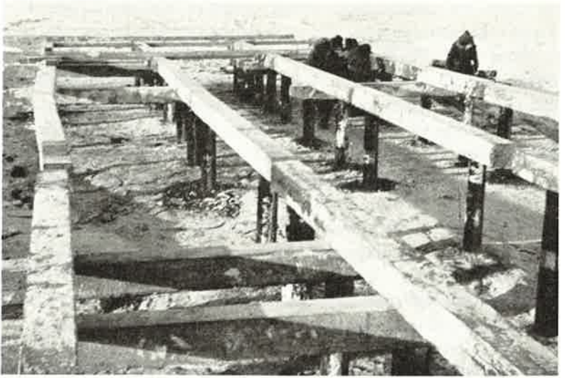
Wood pile foundation.
